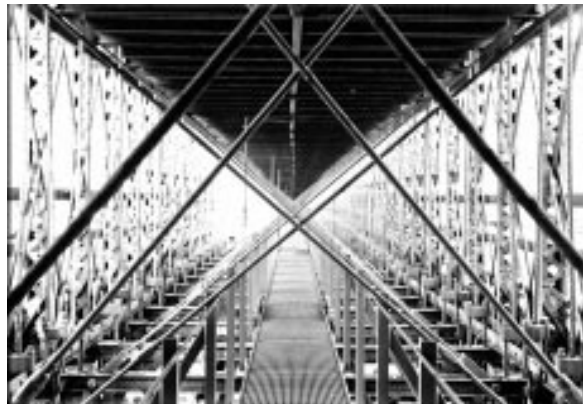
Location of microphones below roadway
