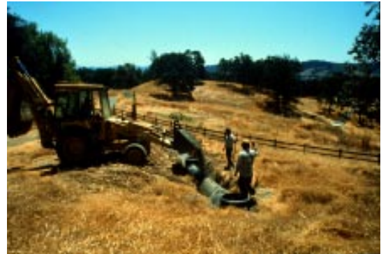
Loudspeaker assembly being buried
