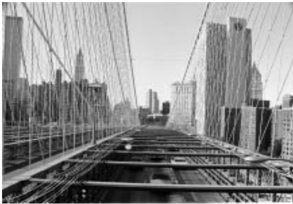
Roadway above bridge facing Manhattan
